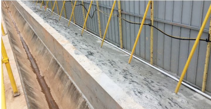
Construct a permanent drain in advance to provide an effective drainage system
