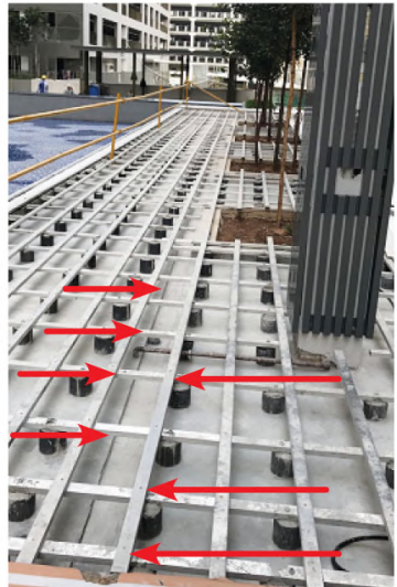
Ground screed to fall and flow test passed before installing timber deck
