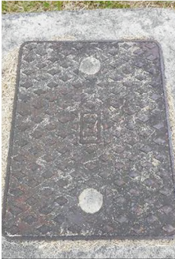
Temporary seal off the lifting point of I/C cover
