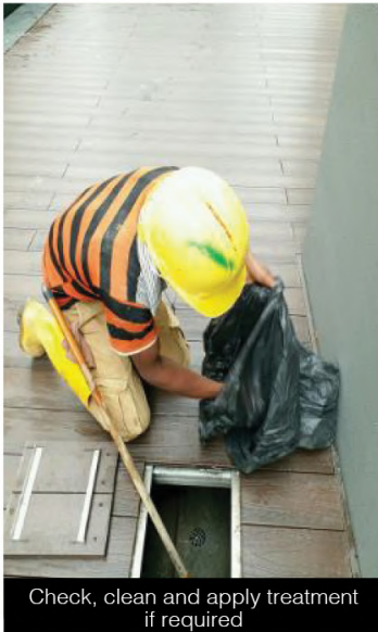
Temporary seal off the lifting point of I/C cover
